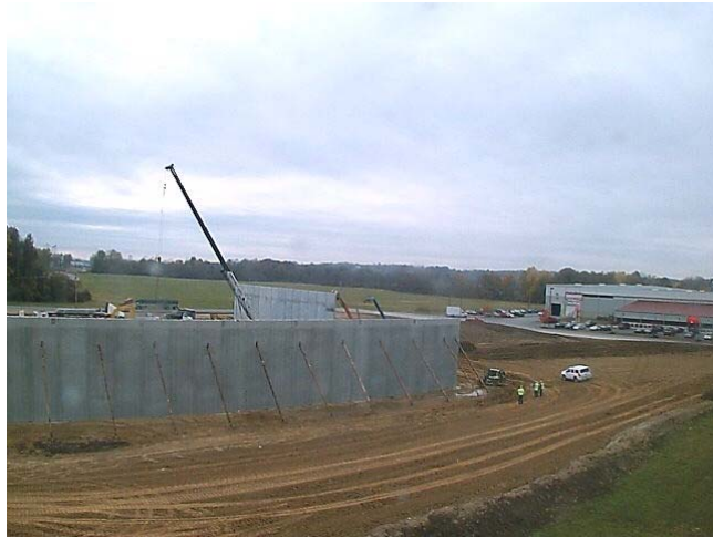
Southgate's new building under construction today
